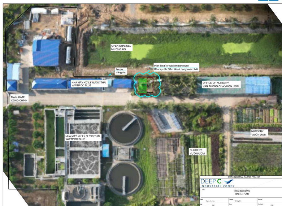
Figure 6. Site of the WWTP in DEEPC IP Hai Phong for the pilot
